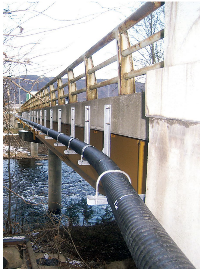
橋梁地覆横曲げ配管
